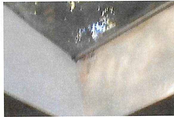
Leak & MOLD IN WINDOW Frame
