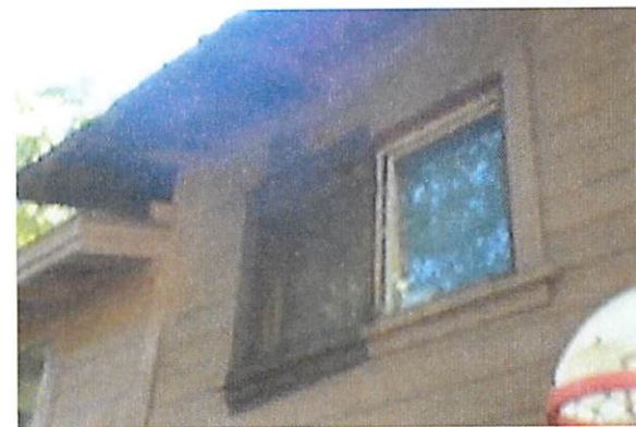
Sealed Screen UNSAFE Egress. from Bed room
